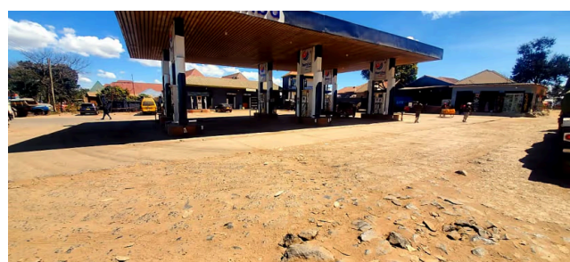
ITEMBA-UZUNGUNI is positioned for corridor traffic along the TANZAM Highway.
